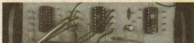
The connections to IC3 and IC4. Note the shorting link at the side of IC3.
